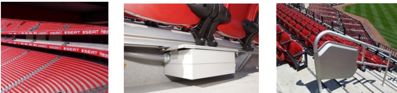
Figure 10: AP1321 under seat or on handrail with NEMA enclosure
